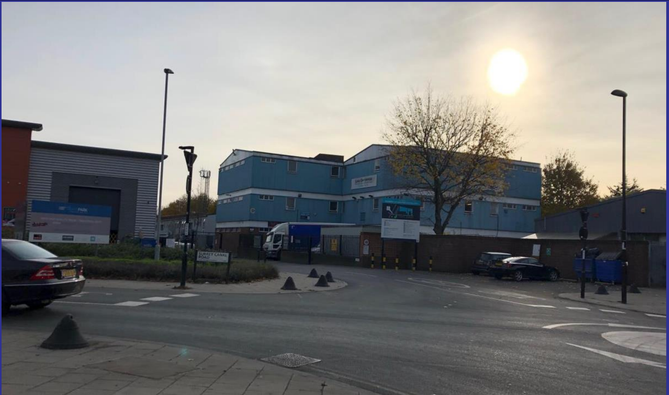
Photograph of existing front and side elevations
