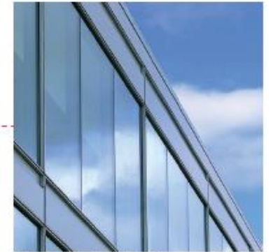
Thermally broken aluminium curtain wall system - RAL 7016
